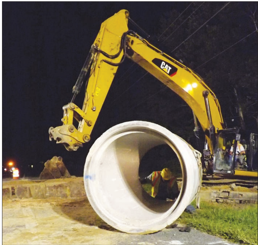
PHOTO COURTESY MARYLAND SHA Construction crews work to install a crossroad pipe as part of the ongoing Route 113 dualization project between Snow Hill and Berlin.
