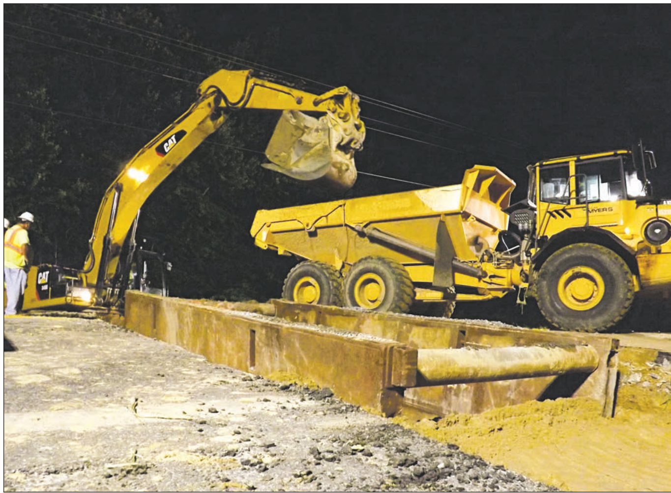
State Highway Administration workers continue to replace stormwater drainage pipes under the road before dualization work can continue. The first batch of four crossings is expected to be complete after Labor Day on Route 113.
