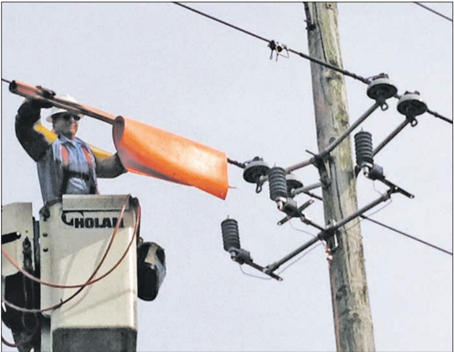
PHOTO COURTESY TIM LAWRENCE Berlin began installing lightning arresters on power lines during the last several months. Arresters absorb lightning strikes and send them to ground, rather than allowing them to travel down power lines and damage infrastructure.
