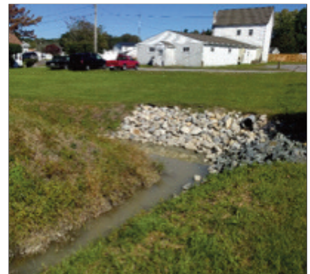
SUBMITTED PHOTO/BAYSIDE GAZETTE Stormwater improvements on Flower Street in Berlin last year included removing accumulated sediment and adding side slope protection to drainage ditches.
