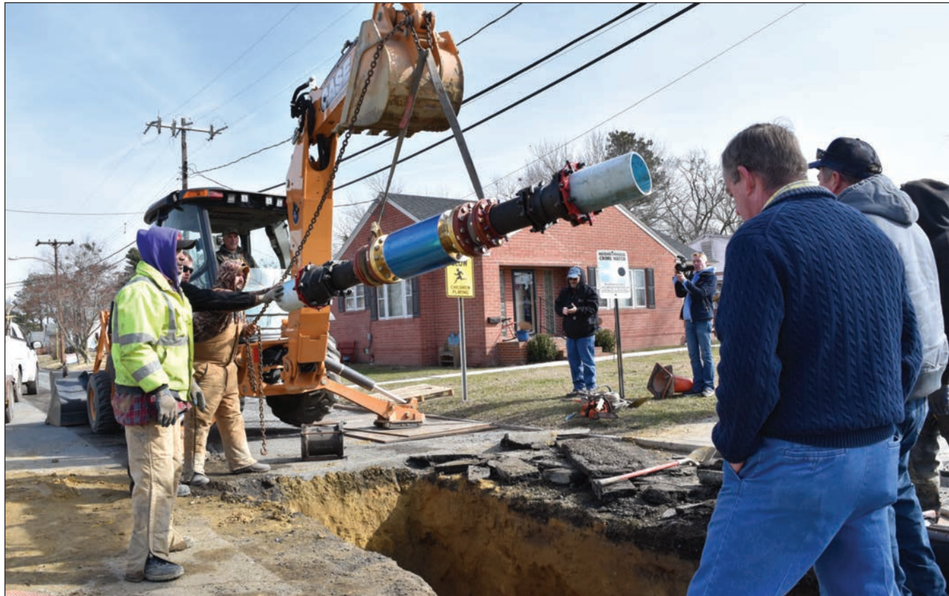
Pocomoke City Public Works, last Friday, install an experimental water-purifying unit near 13th Street and Market Street. The unit, developed by Korean company IOREX, was designed to remove and prevent rust, scale and slime in pipelines using a patented ionization process.
