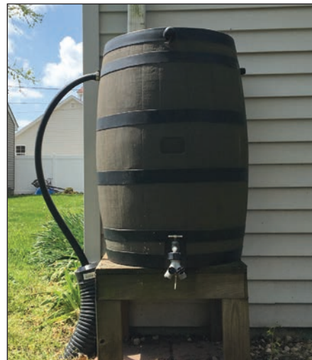
PHOTO COURTESY COLBY PHILLIPS Rain barrels, either DIY or store bought, can reduce excessive stormwater runoff for homeowners and lower pollutants entering area waterways.
