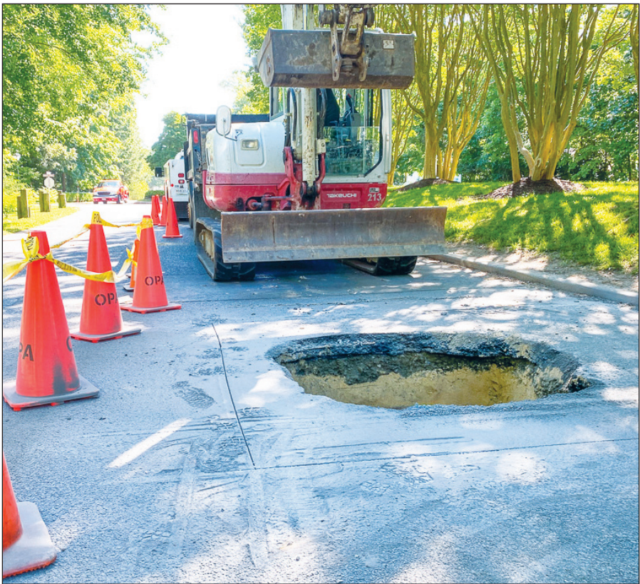
PHOTO COURTESY OCEAN PINES ASSOCIATION Ocean Pines Public Works crews are slated to repair a sinkhole on Mumford's Landing Road this week attributed to prior utility installations.
