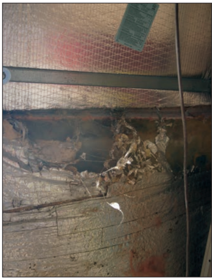
GREG ELLISON/BAYSIDE GAZETTE Remnants of mold inhabiting insulation inside a drop ceiling at the South Station in Ocean Pines.
