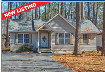
47 FALCON BRIDGE ROAD OCEAN PINES
